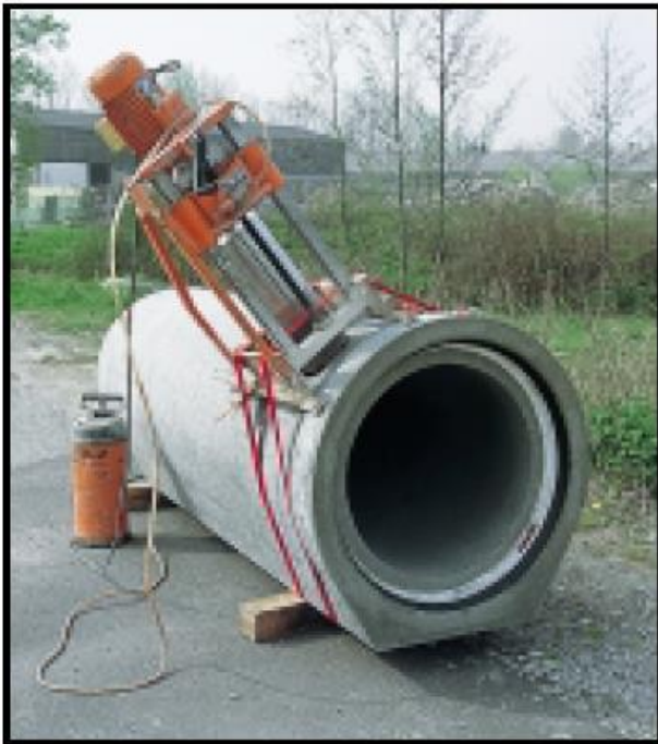
links: Anbohren des FBS-Rohres
