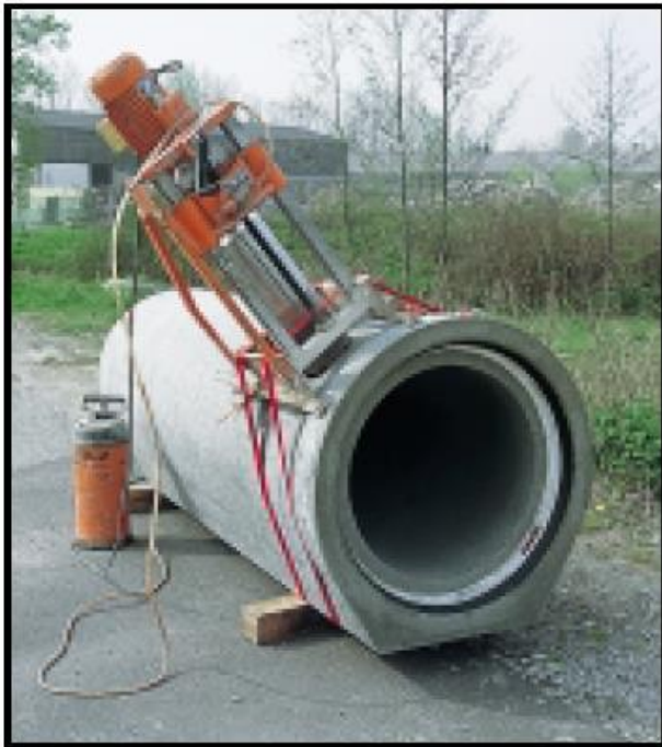
links: Anbohren des FBS-Rohres
